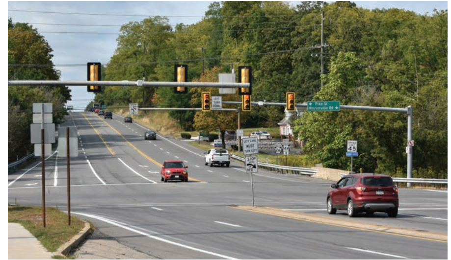
College Avenue intersection with Pike Street and Houserville Road.
