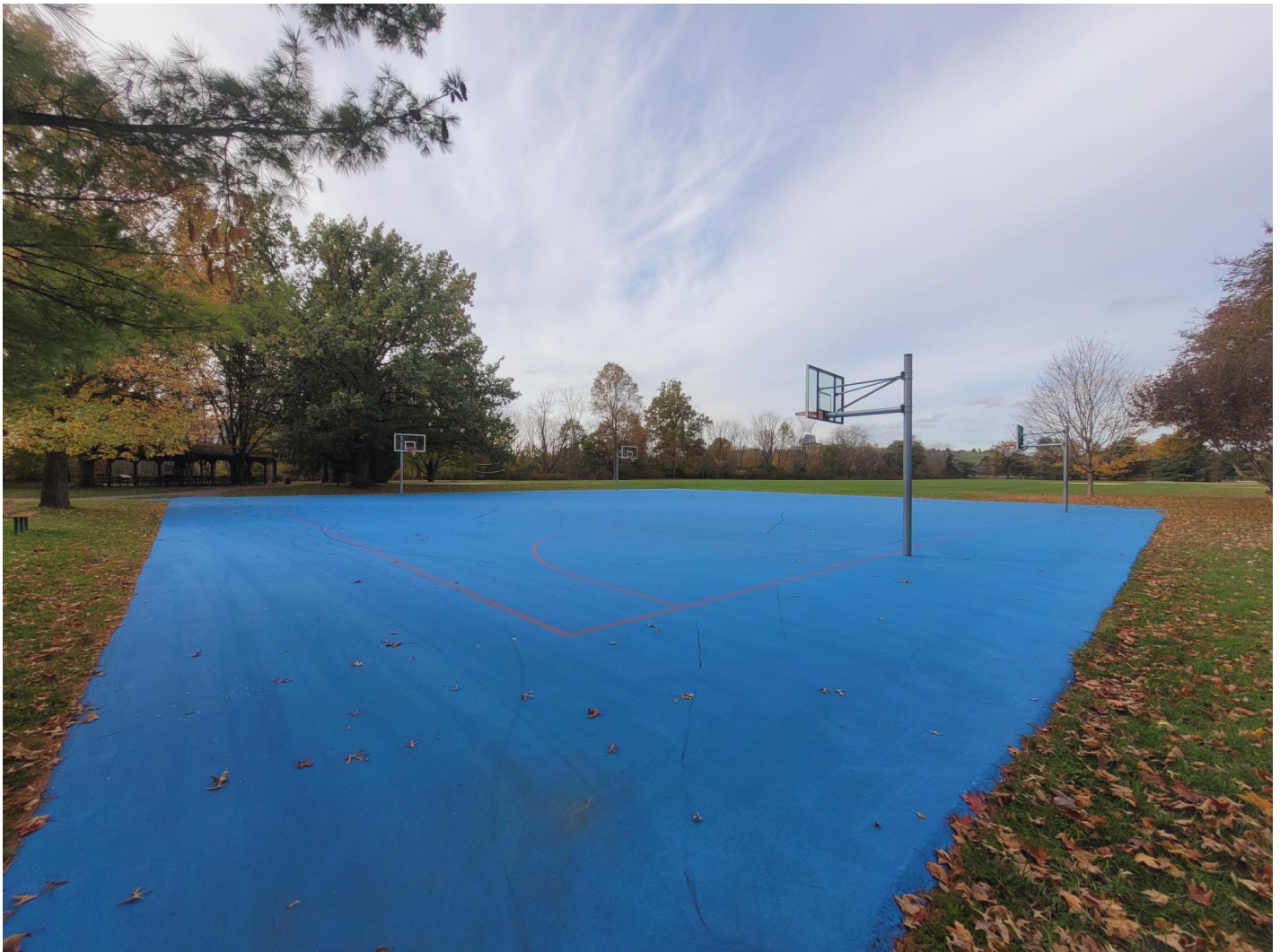
Newly resurfaced basketball court in Spring Creek Park
